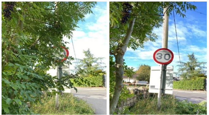
Overgrown vegetation removed in Farmborough
